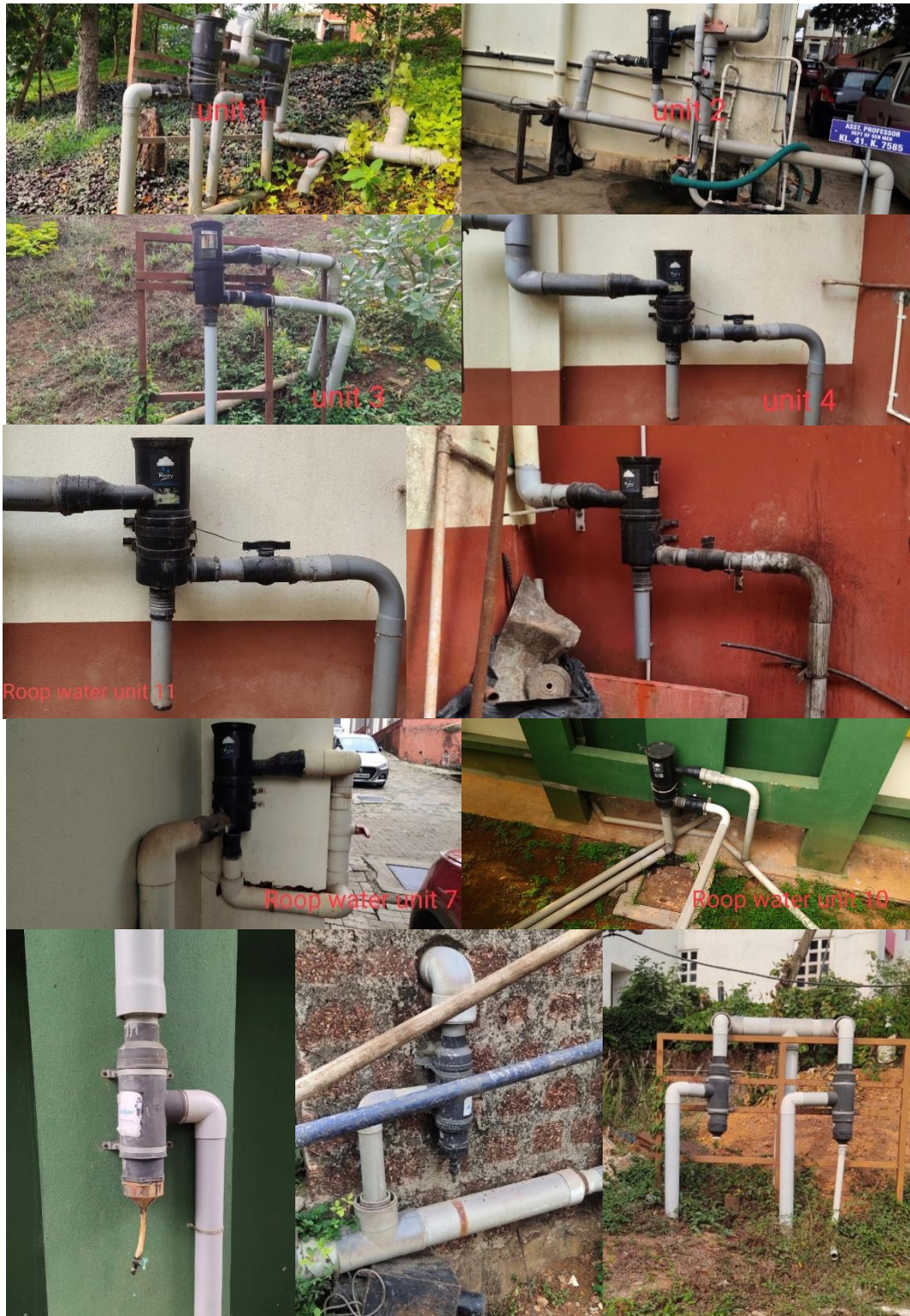
Fig. 23: Roof rainwater harvesting units
