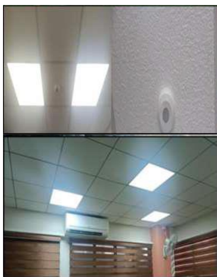
Fig. 29: Sensor for Lighting and LED bulbs
