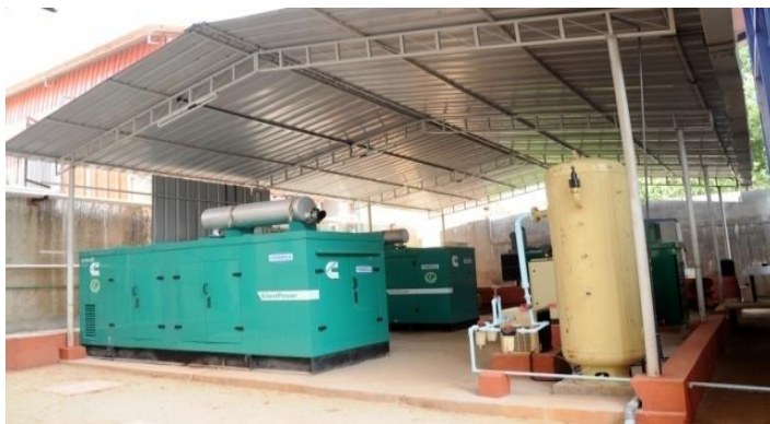
Fig. 13: Diesel Generator
