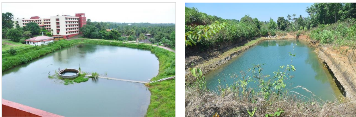
Fig. 22: Rain water harvesting pond
